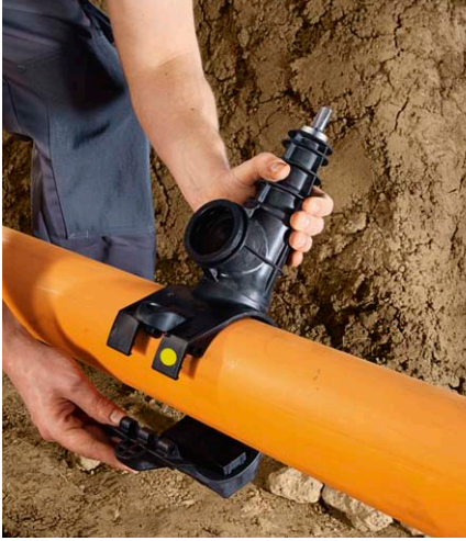
Applying the tapping valve.
