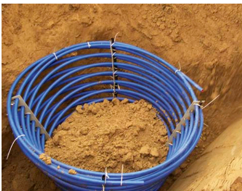
Ground heat baskets capture the heat contained in the upper layers of earth.
