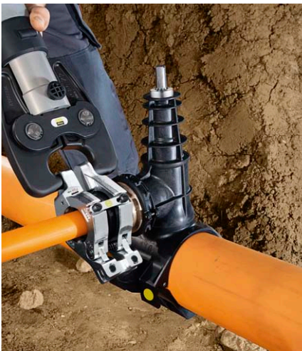
Laying house service connection, pressing and subsequent pressure test.
