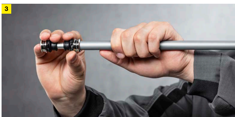
3 Position the connector and check the inspection window.
