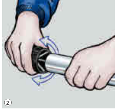
② De-burr pipe internally and externally.
