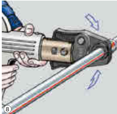
Check the insertion depth and start pressing.
