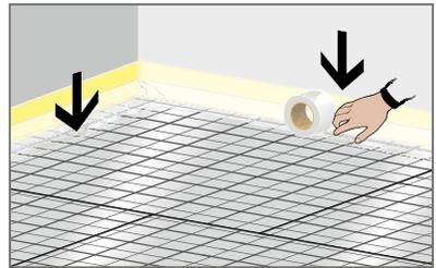
Fig. 104: Fix the foil of the edge insulation strip free of tension on the insulation panels.
