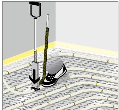
Fig. 106: Lay and staple the heating pipes as marked.
