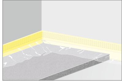
Fig. 72: Lay the footfall sound insulation.
