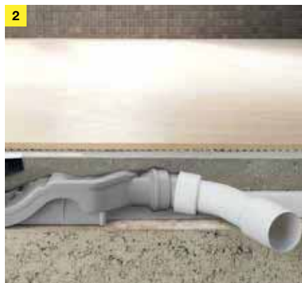
Fig. 2: Extremely flat: The special refurbishment drain reduces the construction height to 70 mm.
